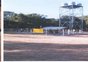
Water Storage Tower
